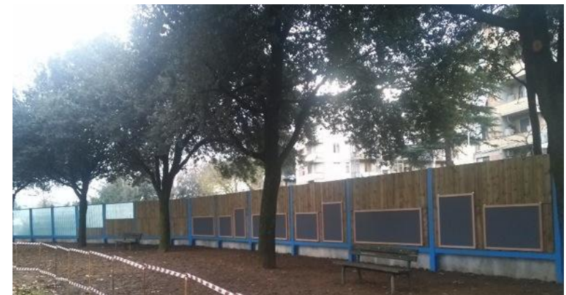
figure 8 Noise barrier at F. Dionisi schoolyard, with integrated blackboards
